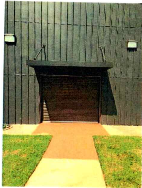
Rear of Building with Garage door
